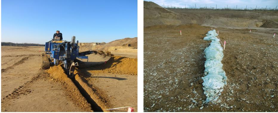
Figure 4: Wheel trench device and injection of geofoam
