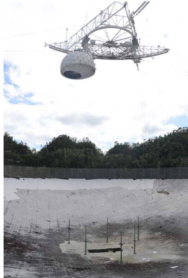
Figure 2.4. The HF antennas in the center of the Arecibo reflector. A wire mesh HF subreflector, not easily resolvable here, hangs under the platform on top of the HF antenna. The sub-reflector altitude is adjusted according to the selected HF frequency.
