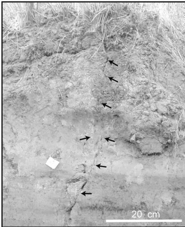
Figure 7. Enlarged photo of eastern wall of trench 1 showing that the crack associated with the youngest event SS1 (outlined by black arrows) appears to extend to the ground surface. We believe this event is the 1990 M_w 5.8 earthquake. See location in Figure 6.
