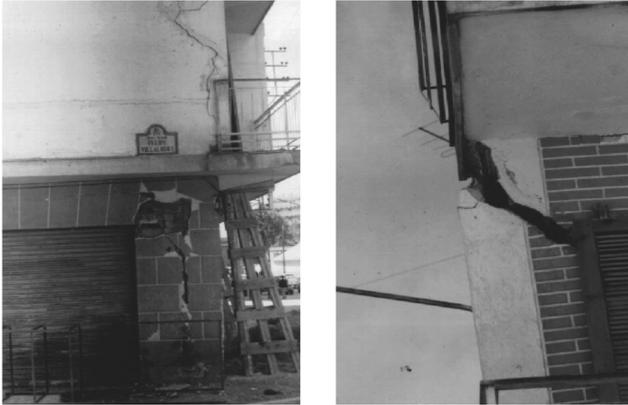
**Fig. 14.** Deterioration in a building in the Calle Pareja Yébenes, which led to the building being evacuated and demolished.
